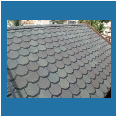
Carriage House Roofing Shingles
