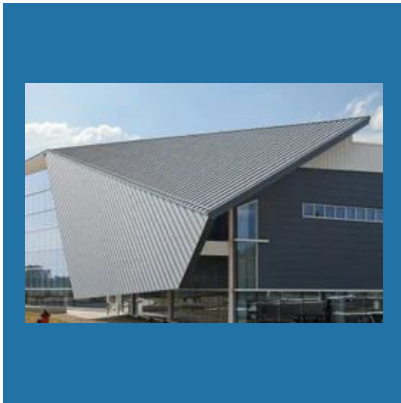
Zinc standing seam roof
